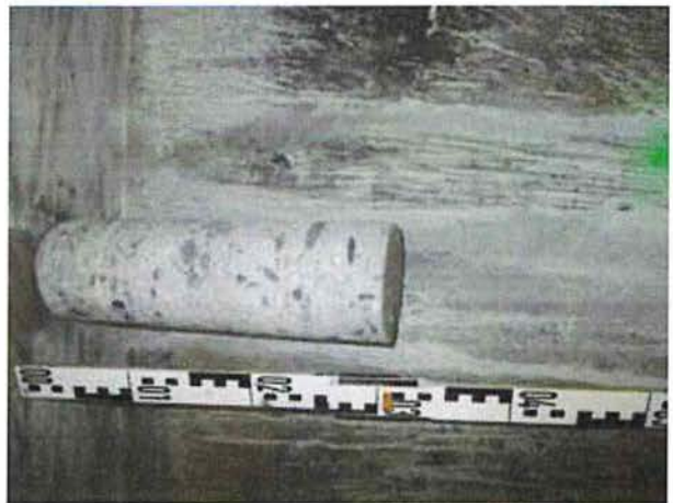
Betonbohrkern KB 5 WP
