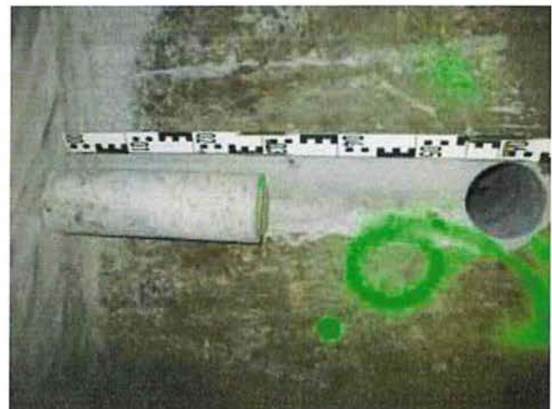
Betonbohrkern KB 6 WP
