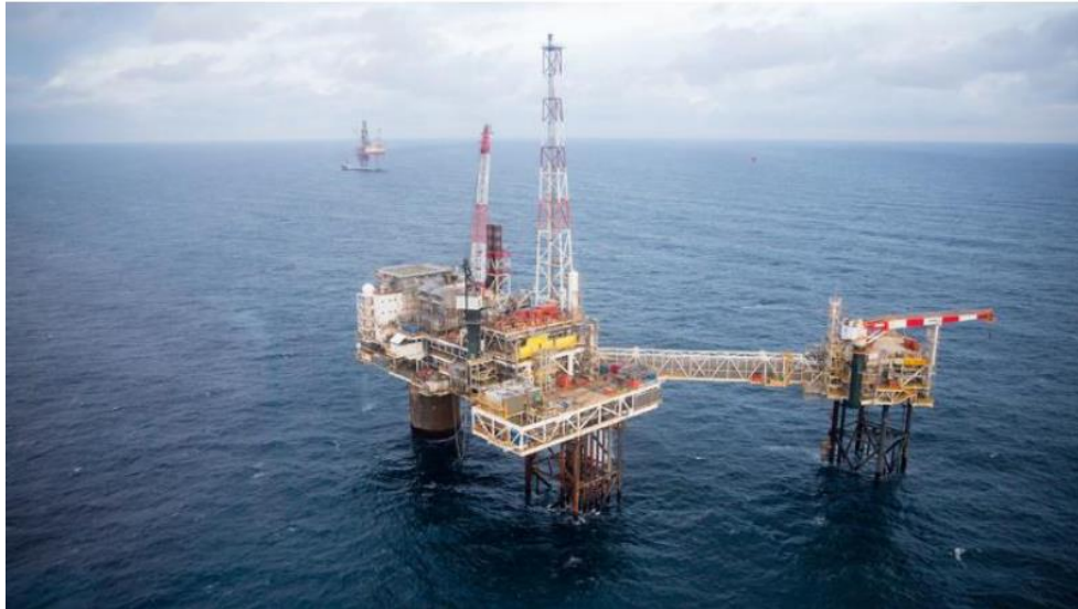
Figure 3-5 South Arne and well head platform East.
