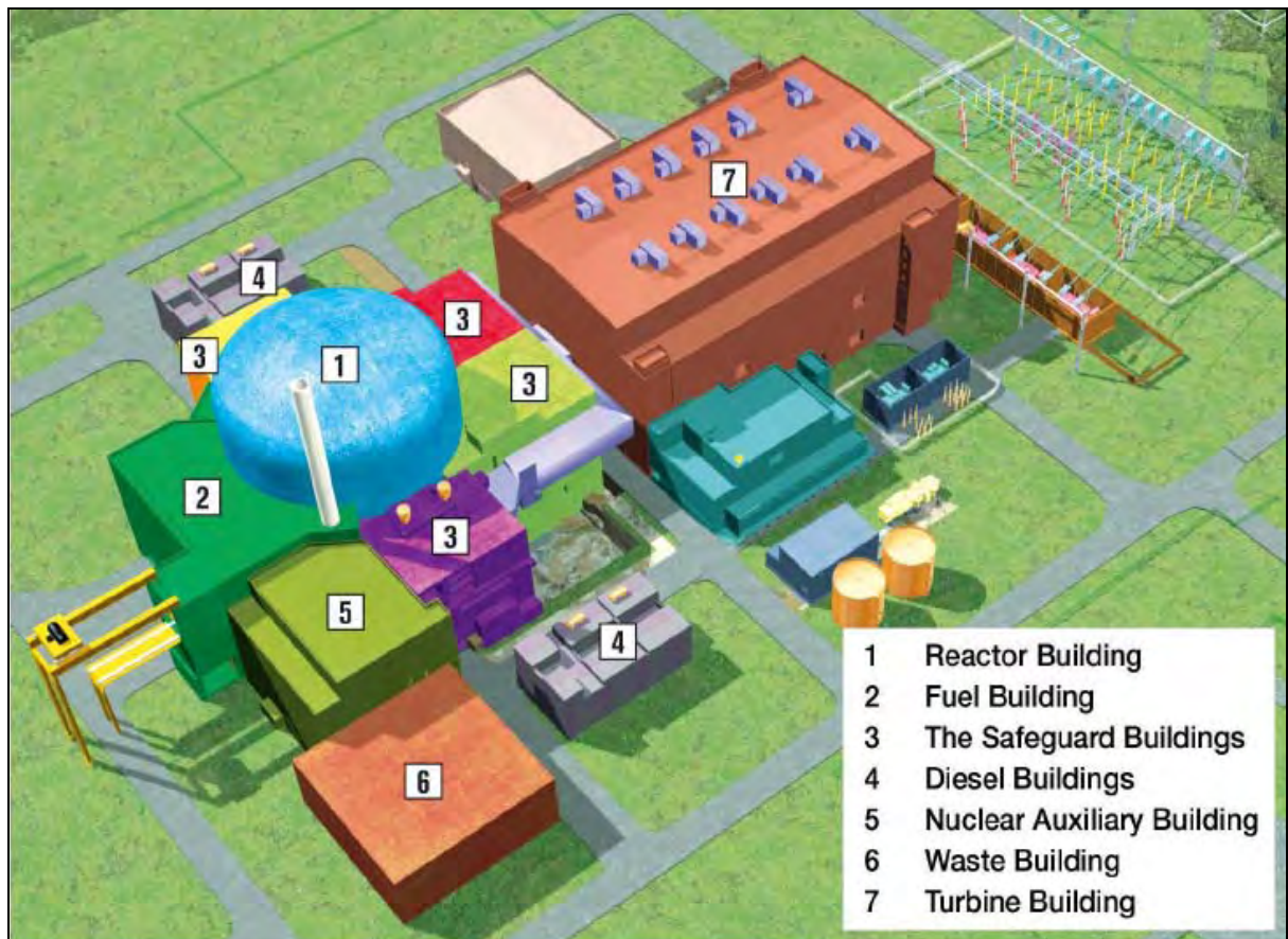
Plate 11F.3: Typical UK EPR plant configuration
