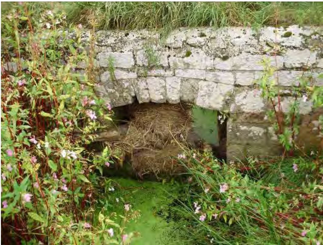
Plates 16.3 and 16.4: Photographs of Holford Stream. The top photo is taken immediately upstream of C182 looking upstream. The bottom photo shows the downstream face of the old sluice where Holford Stream converges with West Brook.
