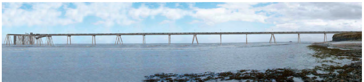
Figure 6.9: View of the Temporary Jetty
