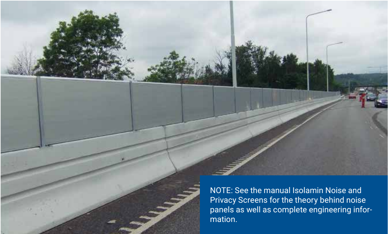
Noise screen along road in central Partille, Gothenburg, Sweden.
