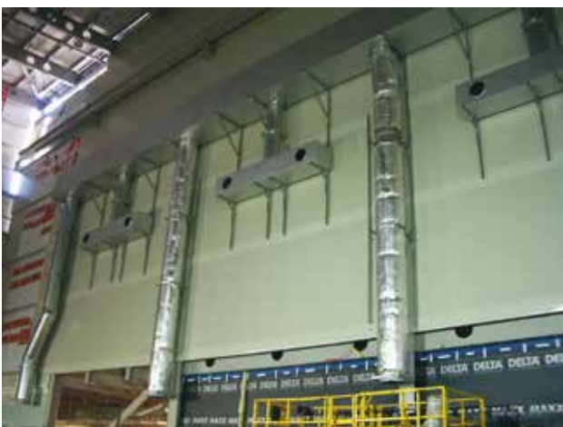
Noise-absorbing firewalls, News International printing press hall, Brouxbourne, England.
